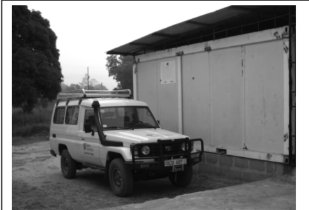
Fig. C. The structure shown, which is adjacent to the KGH laboratory, is constructed from prefabricated office containers donated by the United Nations, which have been subsequently refitted to serve as PCR clean rooms and cell culture suites. A 2006 Toyota Land Cruiser (shown) is available to partly support the proposed project, but will soon require replacement.
