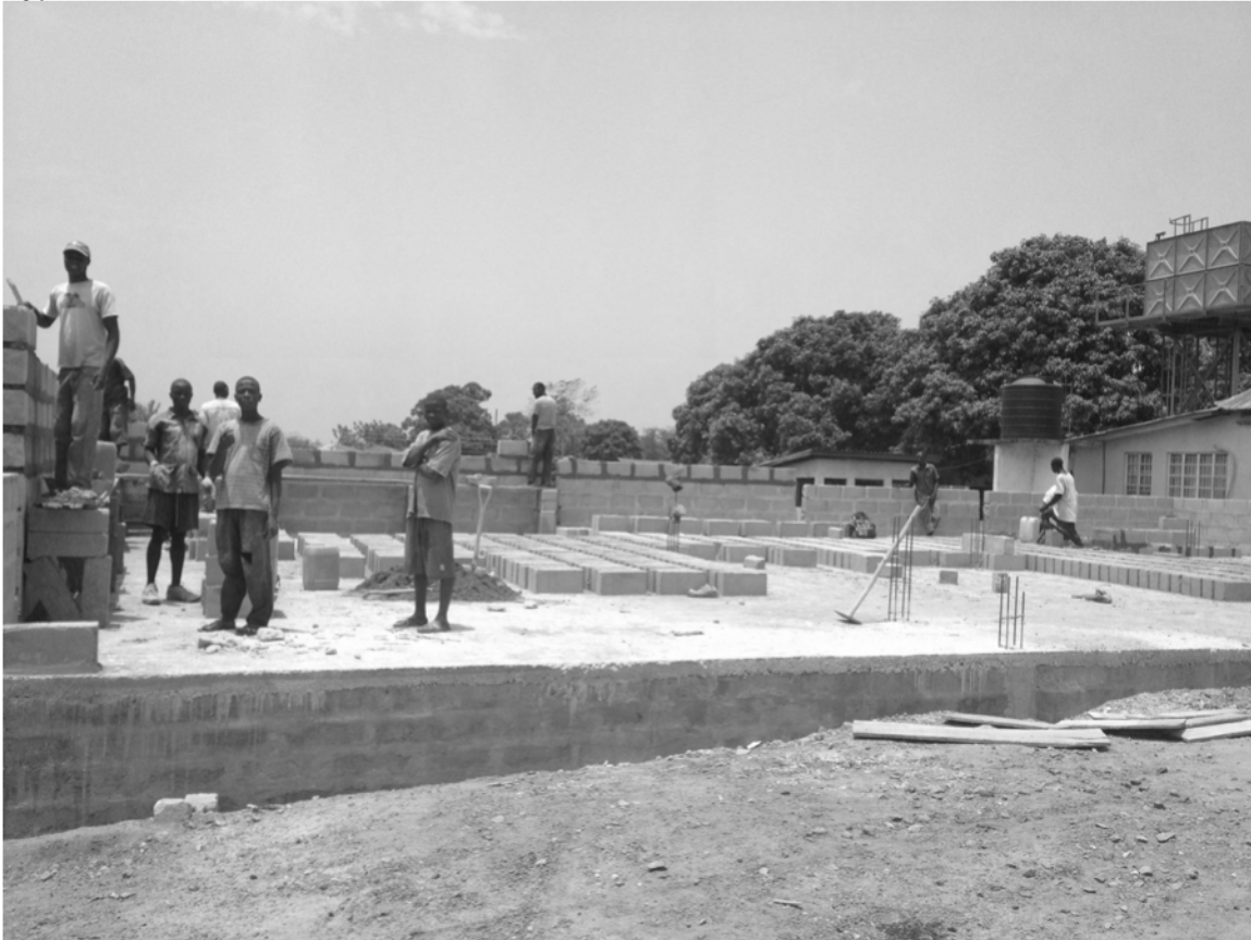
Typical Construction at KGH
