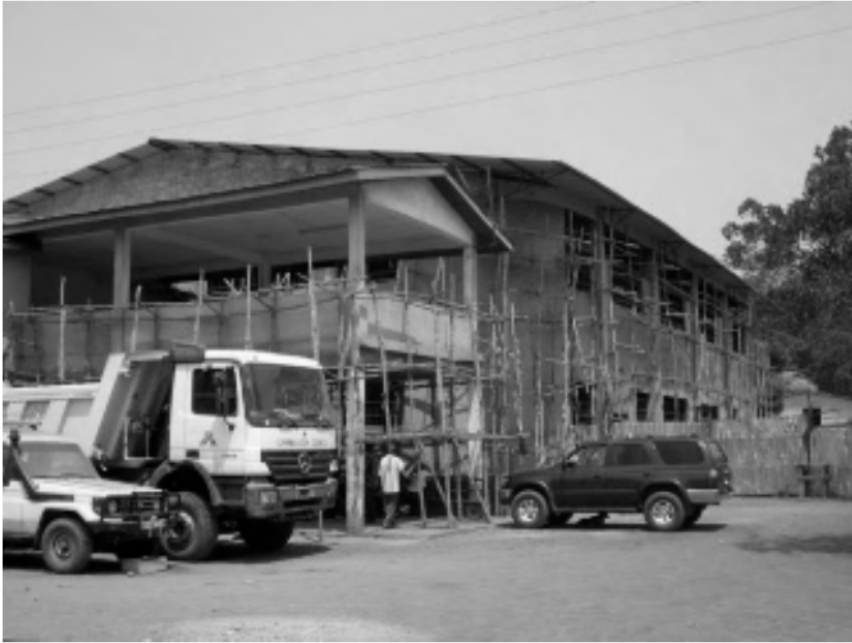
Outside construction of the new hall at Kenema City Council
