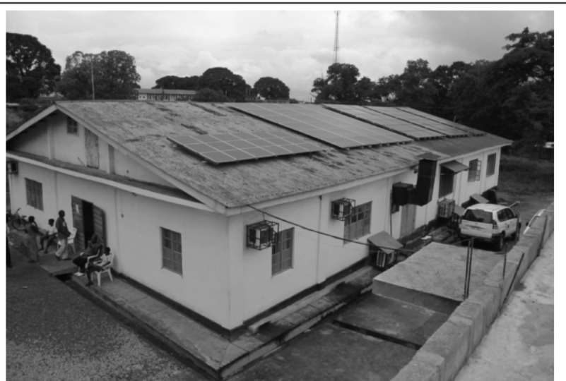
Fig. B. The Kenema Government Hospital Lassa Laboratory. The solar panels provide essential power for refrigerators, freezers and other essential instruments.
