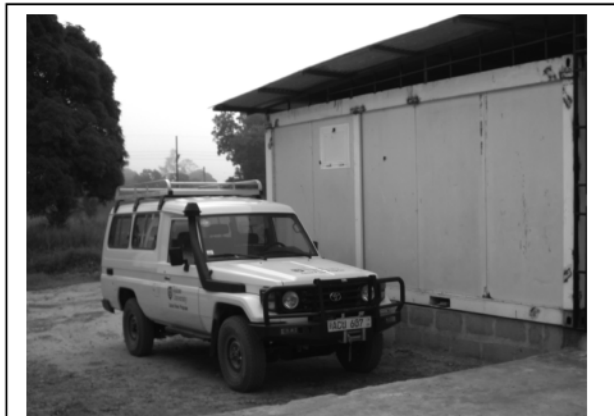
Fig. C. The structure shown, which is adjacent to the KGH laboratory, is constructed from prefabricated office containers donated by the United Nations, which have been subsequently refitted to serve as PCR clean rooms and cell culture suites. A 2006 Toyota Land Cruiser (shown) is available to partly support the proposed project, but will soon require replacement.
